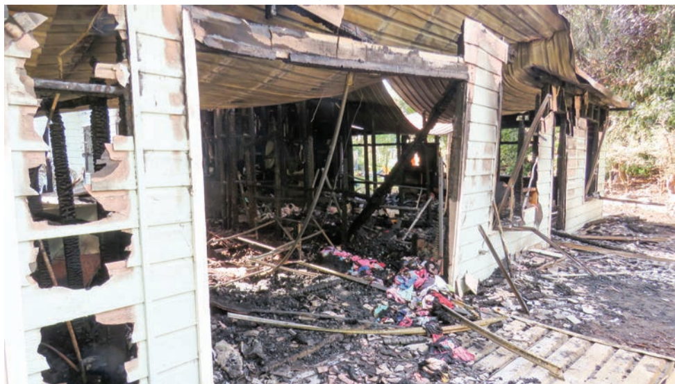
A house in Namu Road was gutted in a fire on Wednesday June 10. See Opunake Fire Service News page 6.
